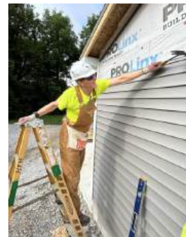
Matthew Smith Nailing Siding
