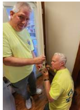
Installing a new door handle - Geary Hoy and Don Smith.
