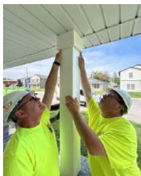
Gene Delaney and Deacon Rob Lortie Installing Front Porch Post
