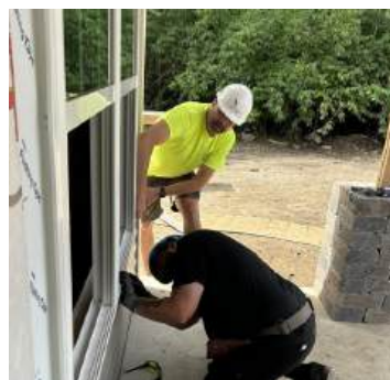
Justin Purdy Installing Siding Under a Window
