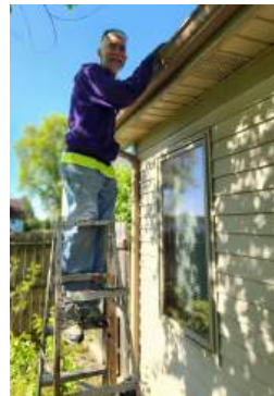
Jim Pifko on gutter detail.
